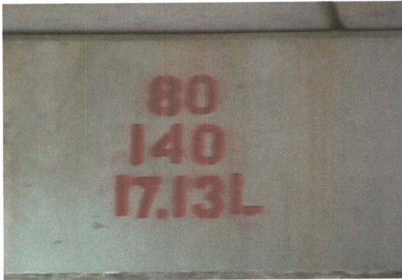
BRIDGE NO. AT ABUTMENT # 1
